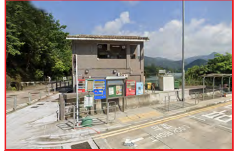
Tai Tam Reservoir (South Gate) 大潭水塘南門開口
